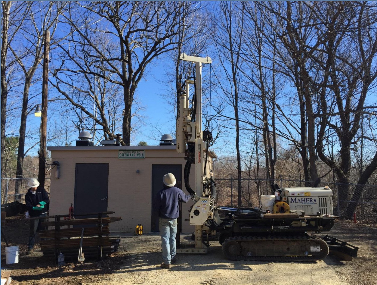
Greenland Well Replacement
