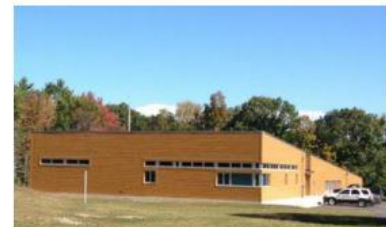
Madbury Water Treatment Facility on Freshet Road
